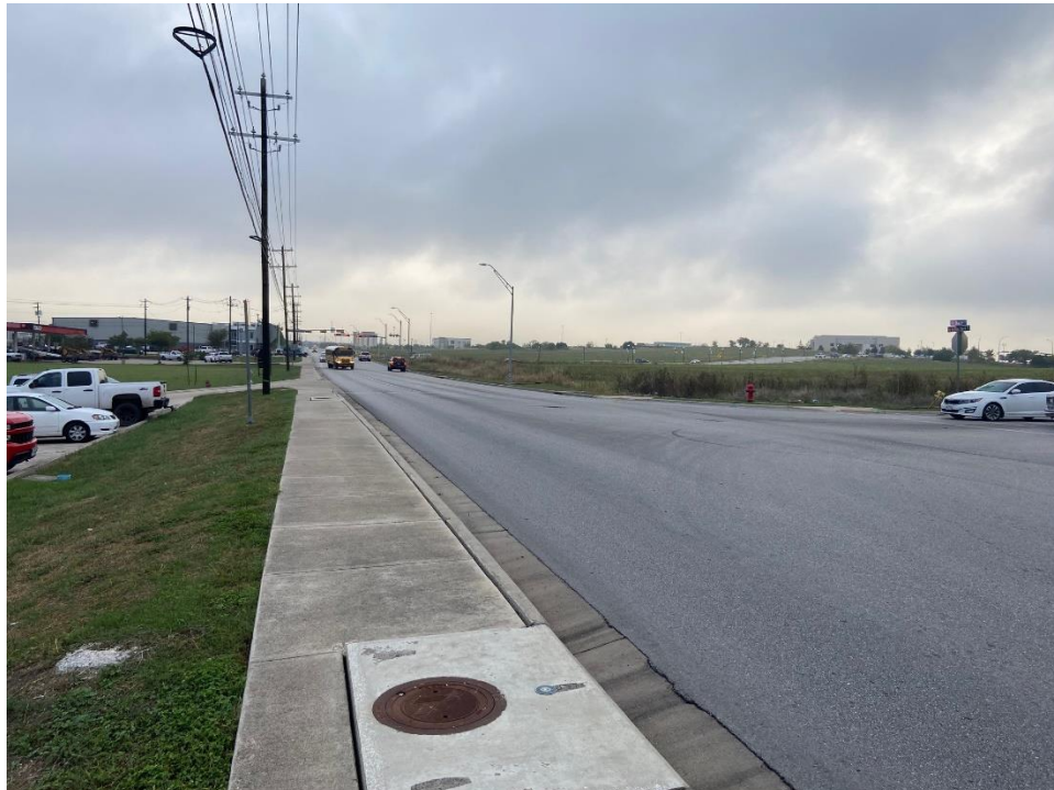
Photo 6: Looking West at Bunton Creek Road and Dacy Lane
