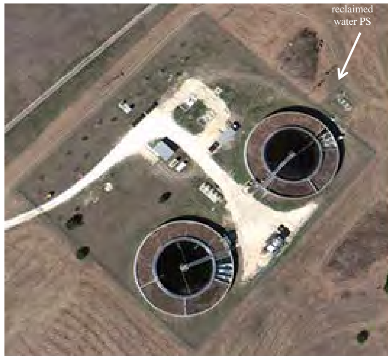
Figure 5-3: Kyle wastewater treatment plant.
