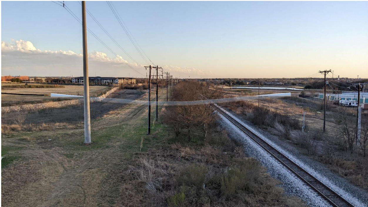
Figure 1 – Railroad Pedestrian Underpass
