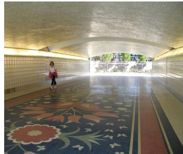
Lighting in an pedestrian underpass should be consistent.
