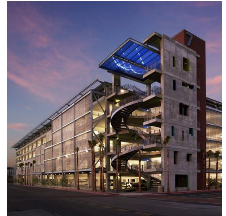
A parking structure can incorporate elements to reduce operational costs, like solar panels.
