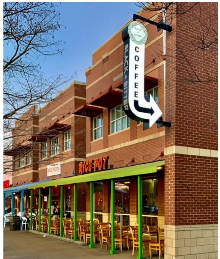
ABOVE: This project provided a new mixed-use building in the heart of downtown Duncanville. The building is designed to frame the street corner with parking behind the building, and includes a mix of office, art, restaurant, and residential spaces.
