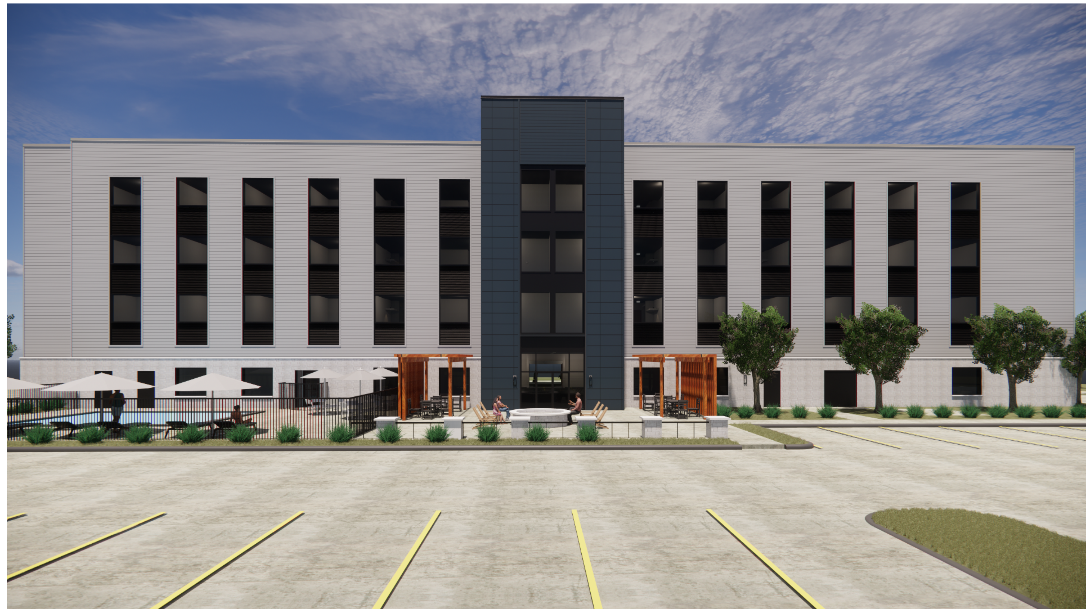
VIEW 1 - EAST FACADE
