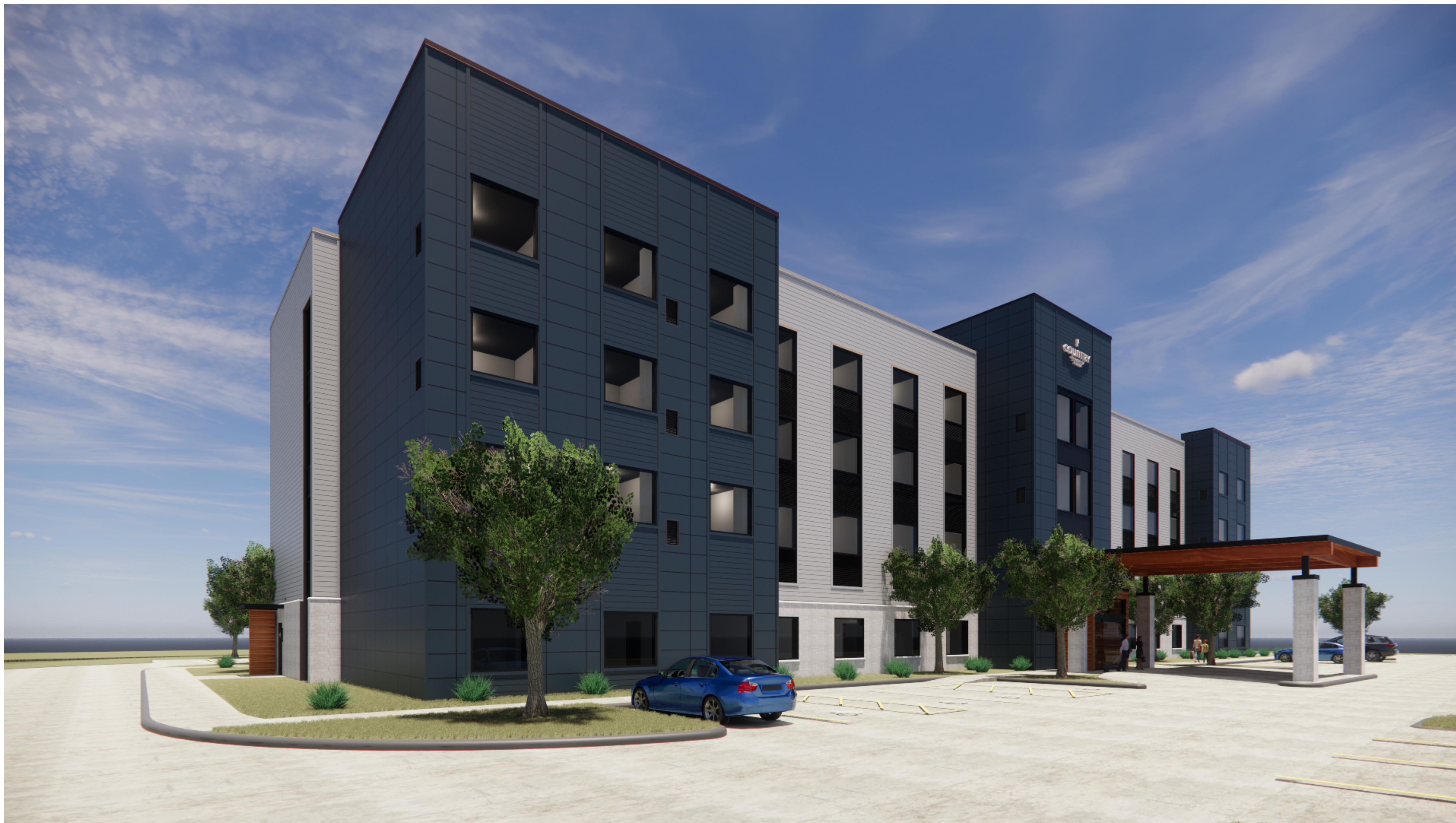
VIEW 2 - NORTHWEST FACADE
