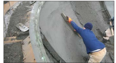
Ecosmart Concrete over crushed recycled concrete sub base
