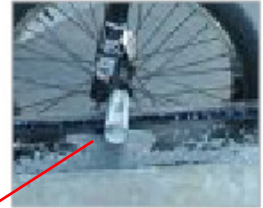
Heavy gauge steel coping back plate protects the bowl deck concrete in Winnipeg
