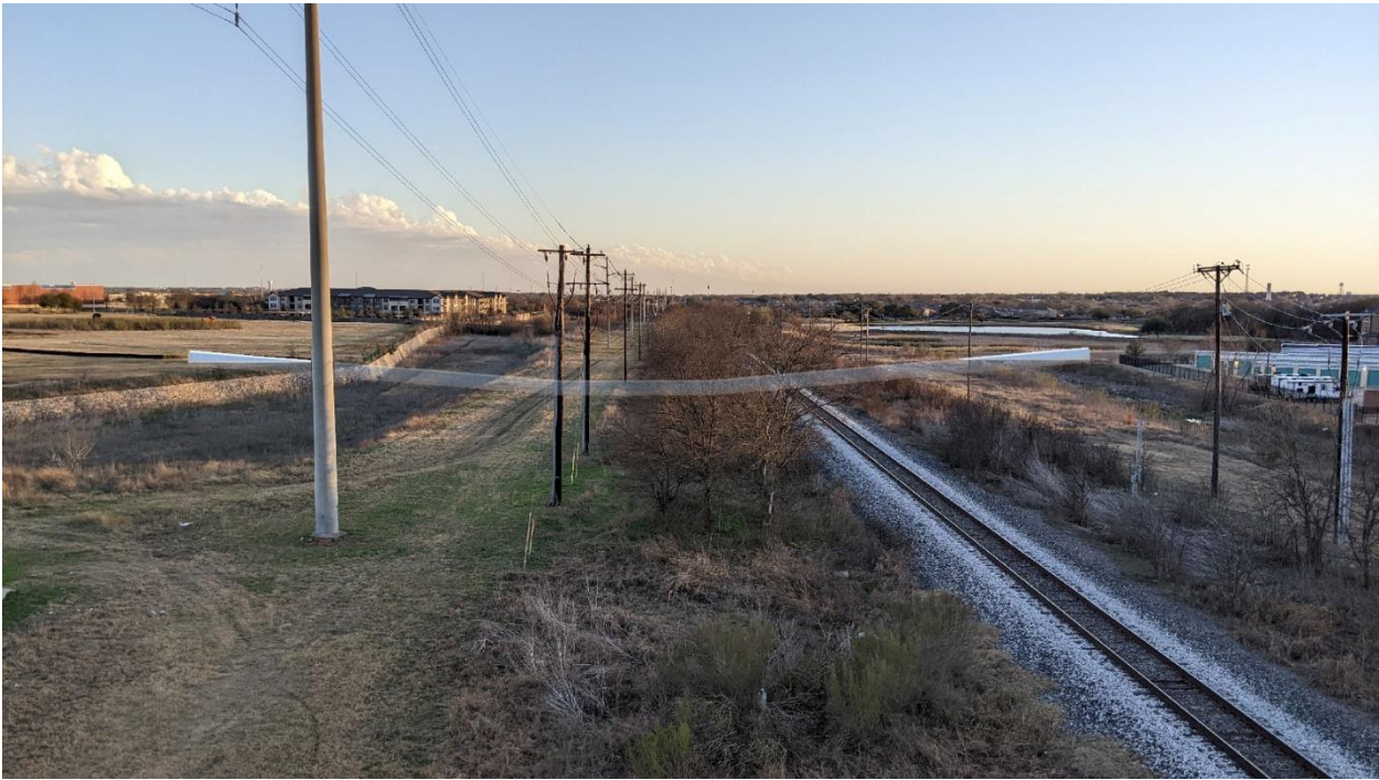
Figure 1 – Railroad Pedestrian Underpass
